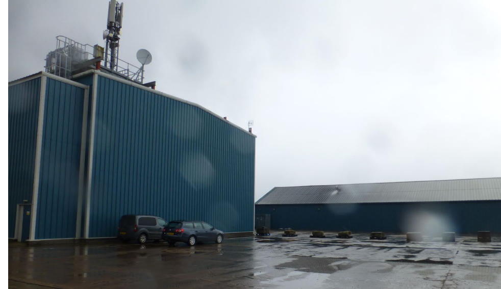
4. View looking east at the location of the proposed new warehouse. Building 26 in on the left; building 25 is in the background.
