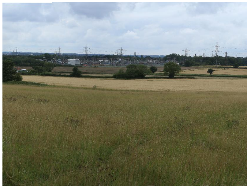
Elstree, London 400kv Substation
