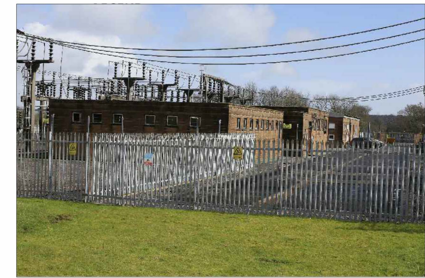
Control Building and Welfare Facilities
