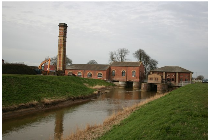
Lade Bank Pumping Station ©Richard Croft
