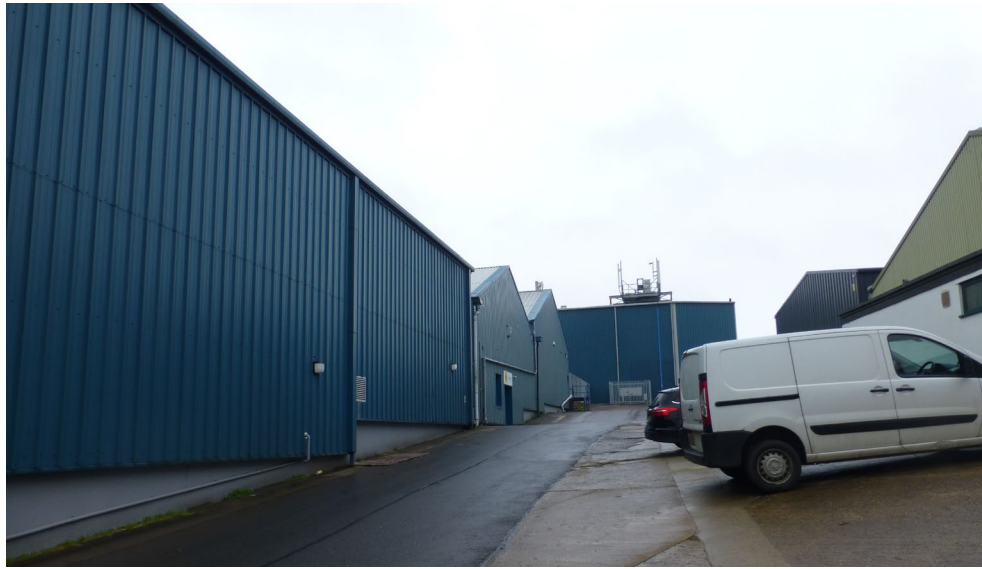
1. View from bottom of internal north road, looking towards building 26. On the left hand side are buildings 36, 25a and 25.
