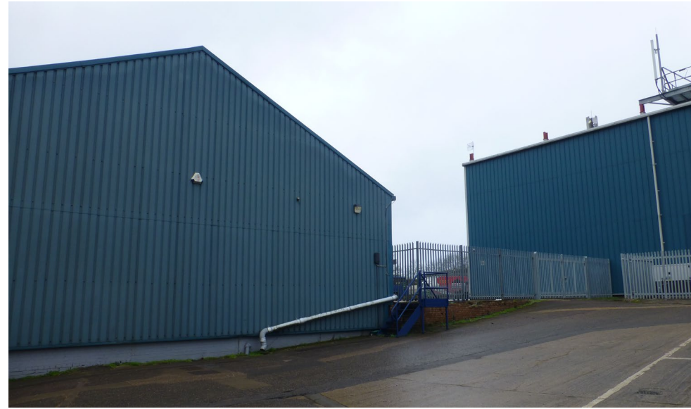
2. View looking west towards the gap between buildings 25 (on the left) and 26 (on the right), where the new warehouse will be located.
