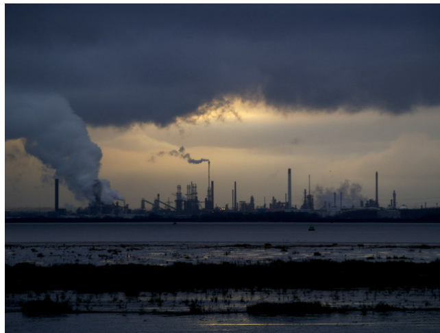
Killingholme Oil Refinery from East Yorkshire © Andy Beecroft
