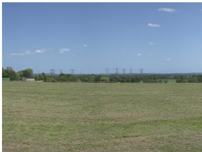
Iron Acton, South Glos 400kv Substation
