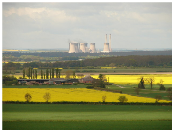
West Burton Power Station © Ian Paterson
