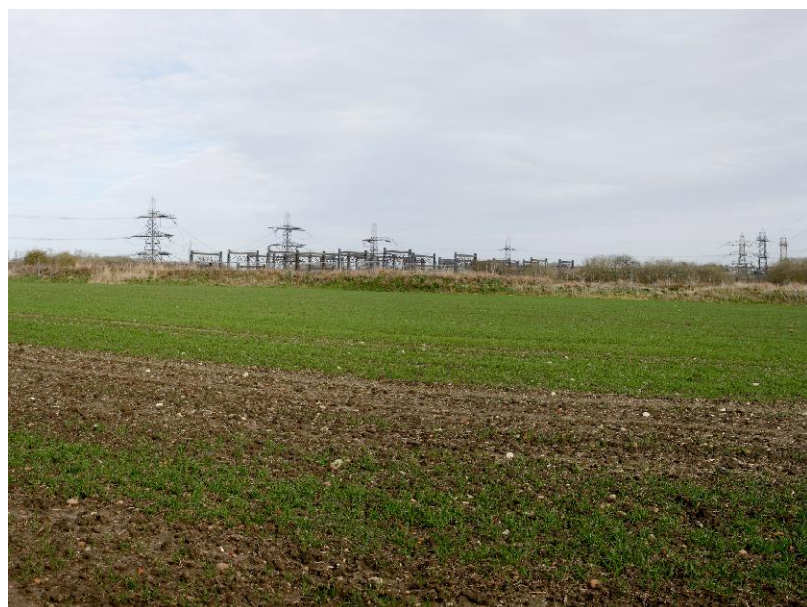
Cowley, Oxford 400kv Substation
