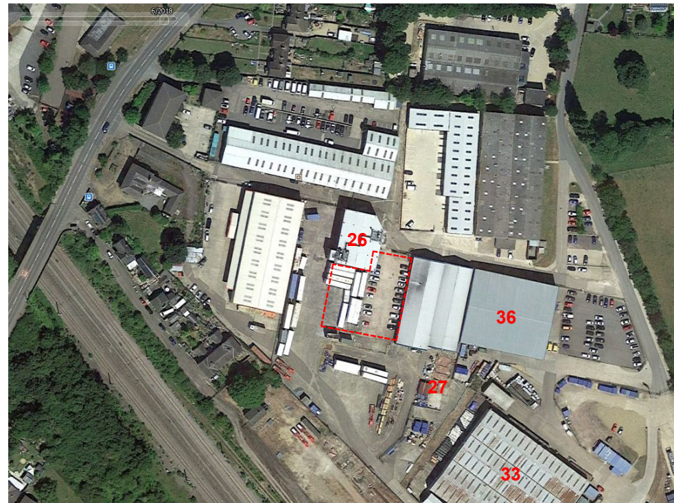
Aerial view © Google Earth Pro - 2018 The view shows demolished building 27, now the location of Bland's coach maintenance workshop.
