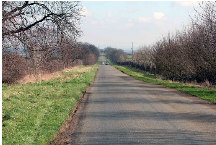
Enclosure Road near Spridlington ©Roger Geach
